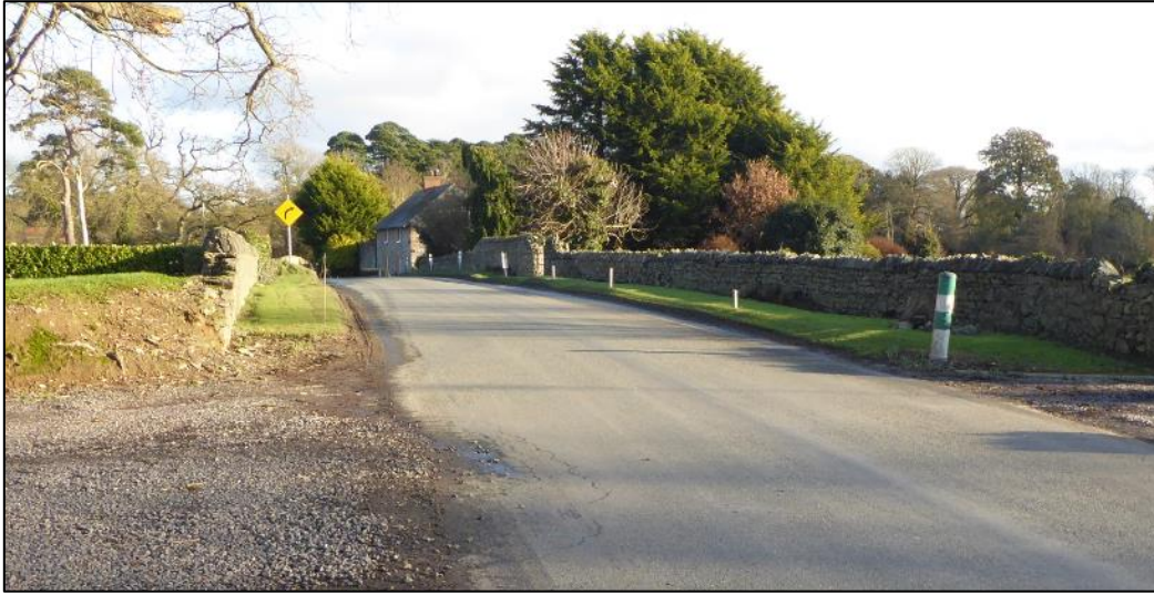
Figure 1-43: Rubble stone walls on approach to Drumcar Bridge on both sides of the road (CH6).
