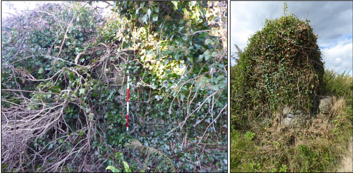
Figure 1-15: Rubble stone boundary wall to Dunany Demesne (RPS LHS019-009).
