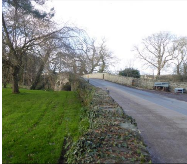
Figure 1-39: Drumcar Bridge (RPS LHS018-052) (looking west).
