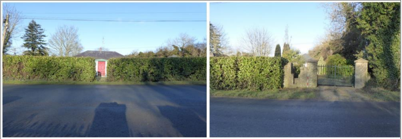
Figure 1-48: Charleville Gate Lodge (CH7) and vehicular entrance.
