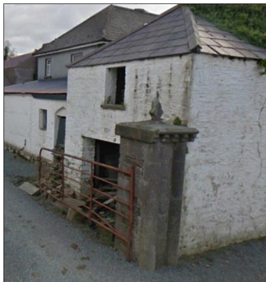
Figure 1-31: CH3, Architectural fragment at the former Post Office in Clonmore.
