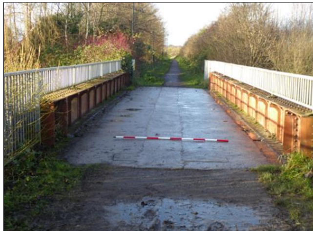
Figure 1-51: Former railway line bridge.
