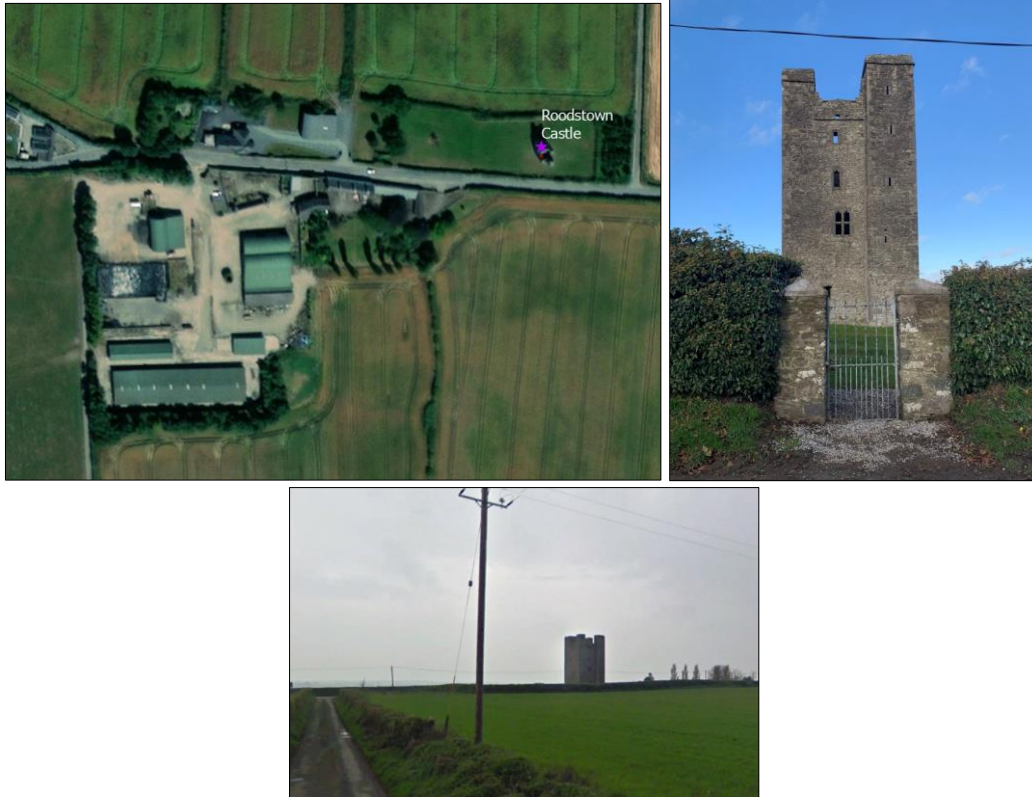
Figure 1-54: Aerial view of Roodstown Castle and the farm buildings to the southeast.
